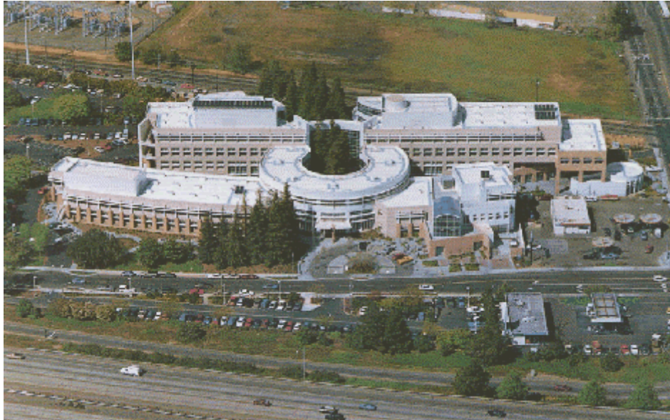
Figure 2: Customer Service Center (CSC) building
