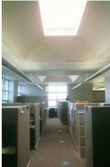
Figure 8: Skylights above work spaces in CSC
