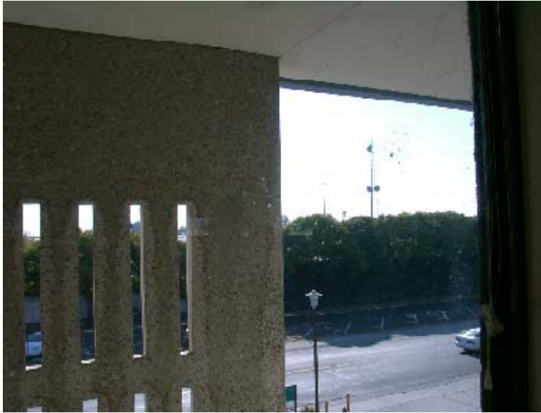
Figure 18: Wide columns blocking view in Distribution Services building.
