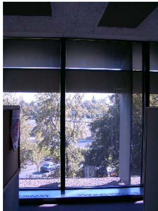
Figure 15: External fins (fixed) on south wall of Headquarters building
