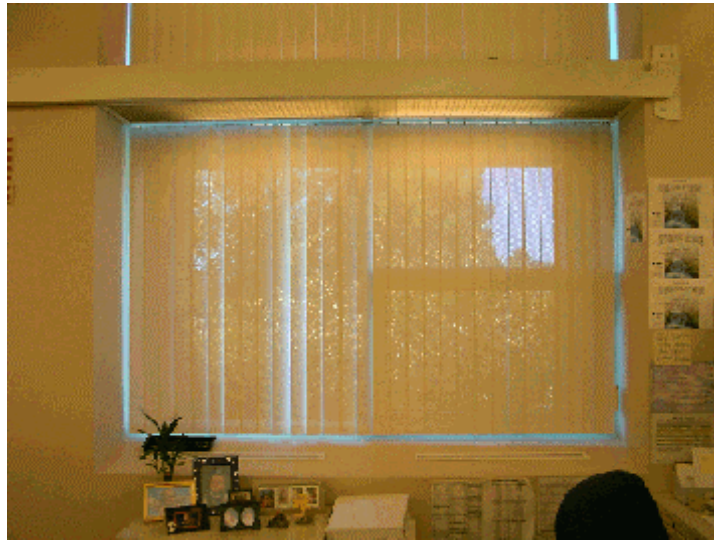
Figure 5: Light shelf with louvered luminaire at south window in CSC building Note partial view through perforated blinds.
