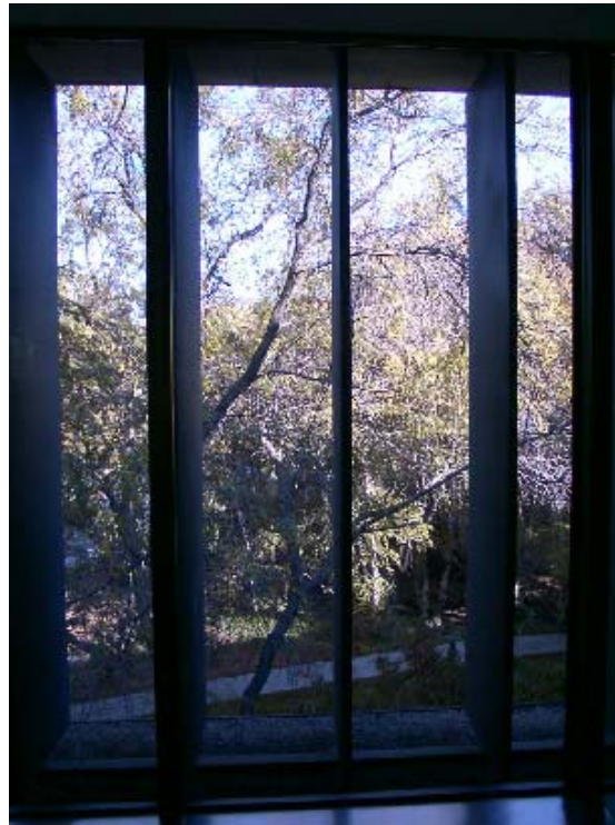
Figure 14: External fins (movable) on east wall of Headquarters building
